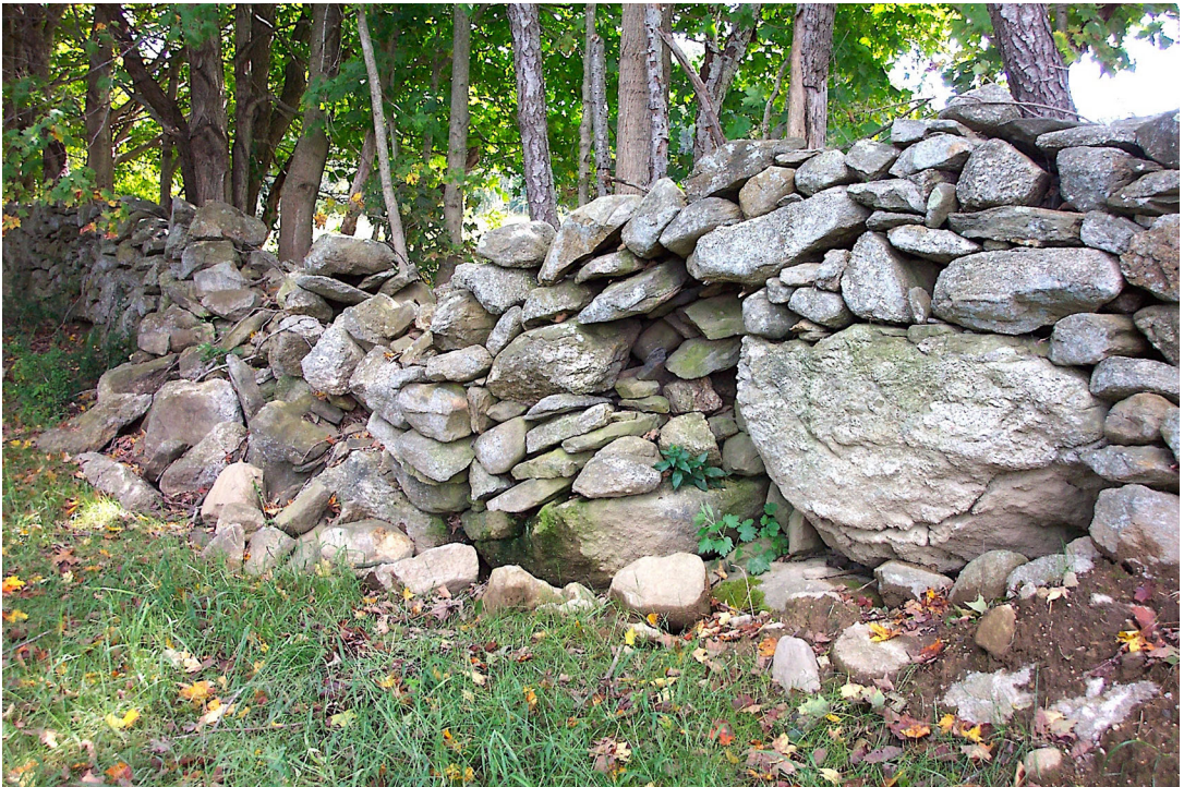
Figure 2. This typical segment of a partially collapsed, single wall in Hebron, Connecticut, shows a range of stone sizes, a variety of lithologies, a stacked degree of order, no mortar, and a single tier with no courses. These terms are part of the nomenclature for an emerging stone wall science that is undergirding stone wall inventory, management, and interpretation. (Photo by author)
