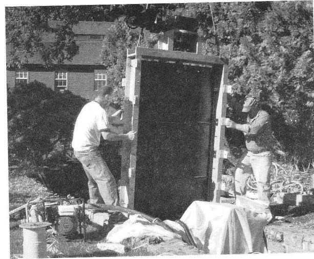
Will Davidson and John Mahan, workers for Machnik Bros, guide the new water control gate into place.
