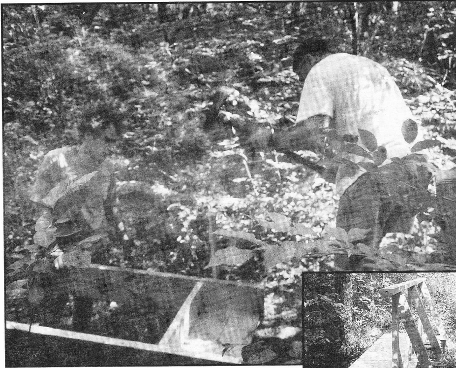
Ralph Lewis and Anthony Irving installing a new bridge at the entry to the Pleasant Valley Preserve. It is made of Enviro Board, a recycled plastic material used by the Forest Service. It is long lasting, looks like wood, but does not have the adverse environmental effects of pressure treated wood.
