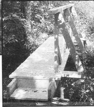
Ralph Lewis and Anthony Irving installing a new bridge at the entry to the Pleasant Valley Preserve. It is made of Enviro Board, a recycled plastic material used by the Forest Service. It is long lasting, looks like wood, but does not have the adverse environmental effects of pressure treated wood.
