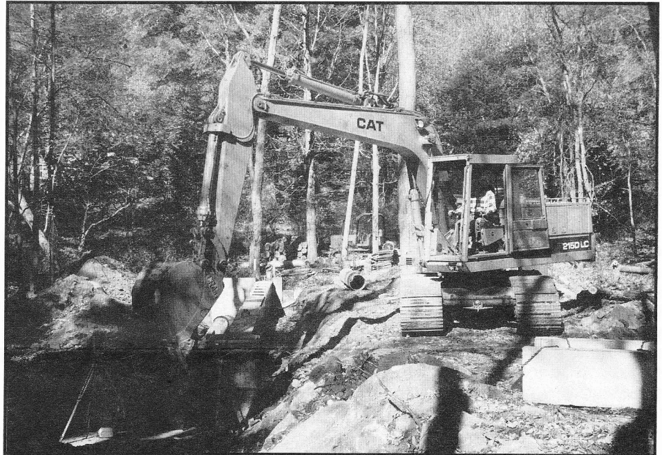
Digging to install fish ladder.
