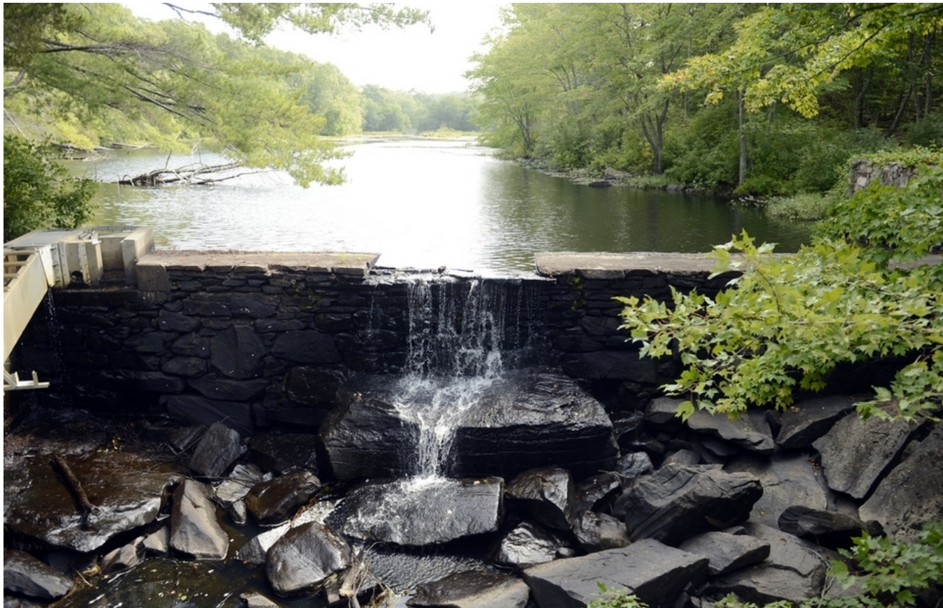
The Ed Bill's Dam on the Eight Mile River in Lyme Friday, Sept. 4, 2015. Demolition of the dam, one of if not the last on the river, will begin September 14th. (Sean D. Elliot/The Day)
